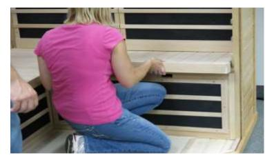
The Bench Top should fit down flush from front to back. It may be necessary to use the
